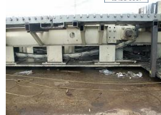
Blank de-stacker Blow line_Nartech, Guelph
